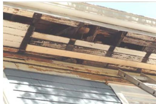
Water damage under the eaves on the south side.
